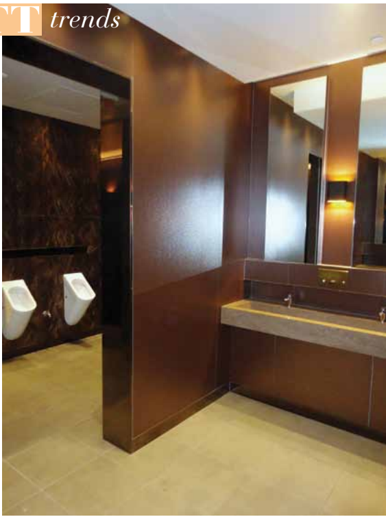
3 & 4. Large 300 x 100 cm panels of Laminam recently installed at Star City Casino, Sydney.
