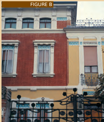
FIGURE B CLOSE TO THE POLETTA HOME IN FERRARA IS THIS ELEGANT 'STILE LIBERTY' VILLA WITH CERAMIC TILES SET INTO THE FACADE; THEIR SINUOUS LINES ECHOED IN THOSE OF THE WROUGHT IRON GATE AND BALCONY.
