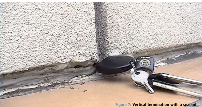
Figure 7: Vertical termination with a sealant.
