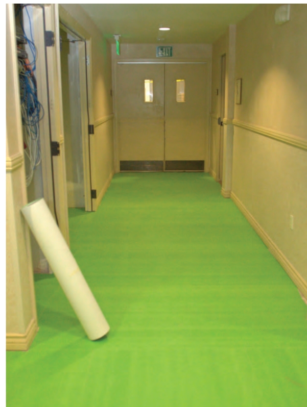
Right: Surface cracks usually appear in new concrete within 12 months of the screed being poured. The entire floor can be covered with an anti-fracture membrane like the featured GreenSkin, which can also be used effectively to isolate individual cracks. (Images courtesy of CDK Stone.)
