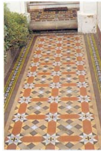
Tessellated path and verandah, Sydney suburb of Annandale. Note the encaustic flowers in the border.
