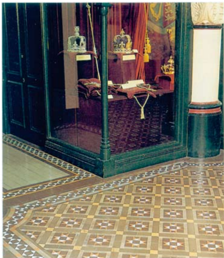
One of the restored floors in the Queen Victoria Building, Sydney
