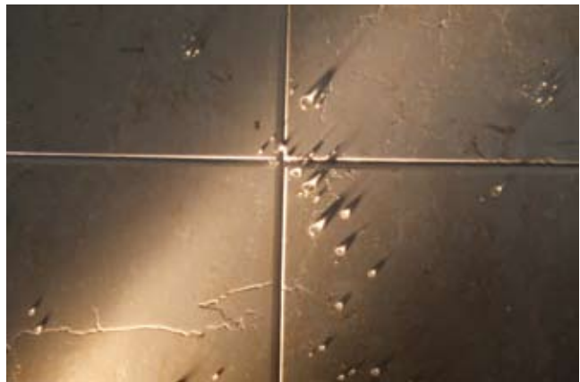
Photo 4. The application of a penetrating sealer prevents or minimises water penetration through the tiles and grout.
