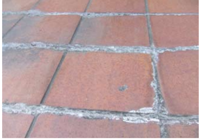
Photo 2. Efflorescence forming where moisture below the impervious tiles rises through cracks in the grout.
