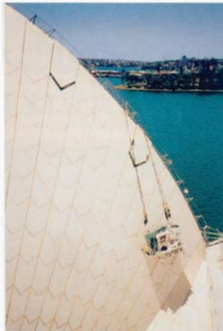
Special carriages allow two crews to inspect individual "Tile Lids"
