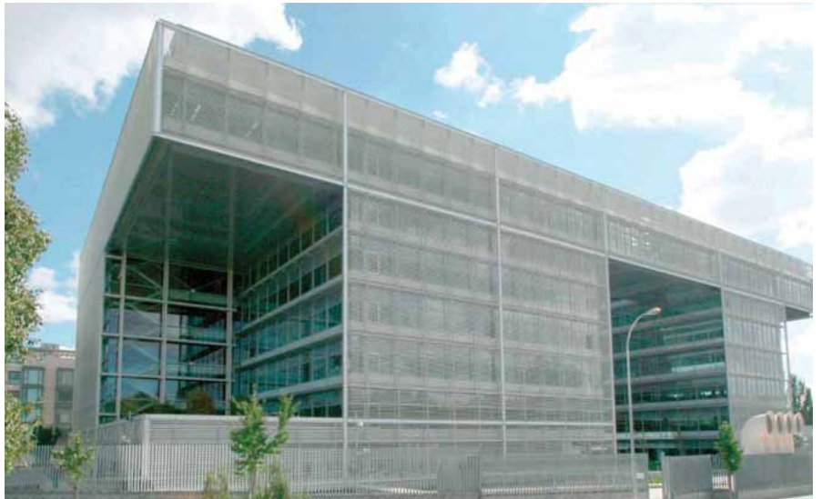
New Banco Popular headquarters designed by Ayala Architecture features a ventilated facade made from extruded stoneware (ceramic) cylinders.
